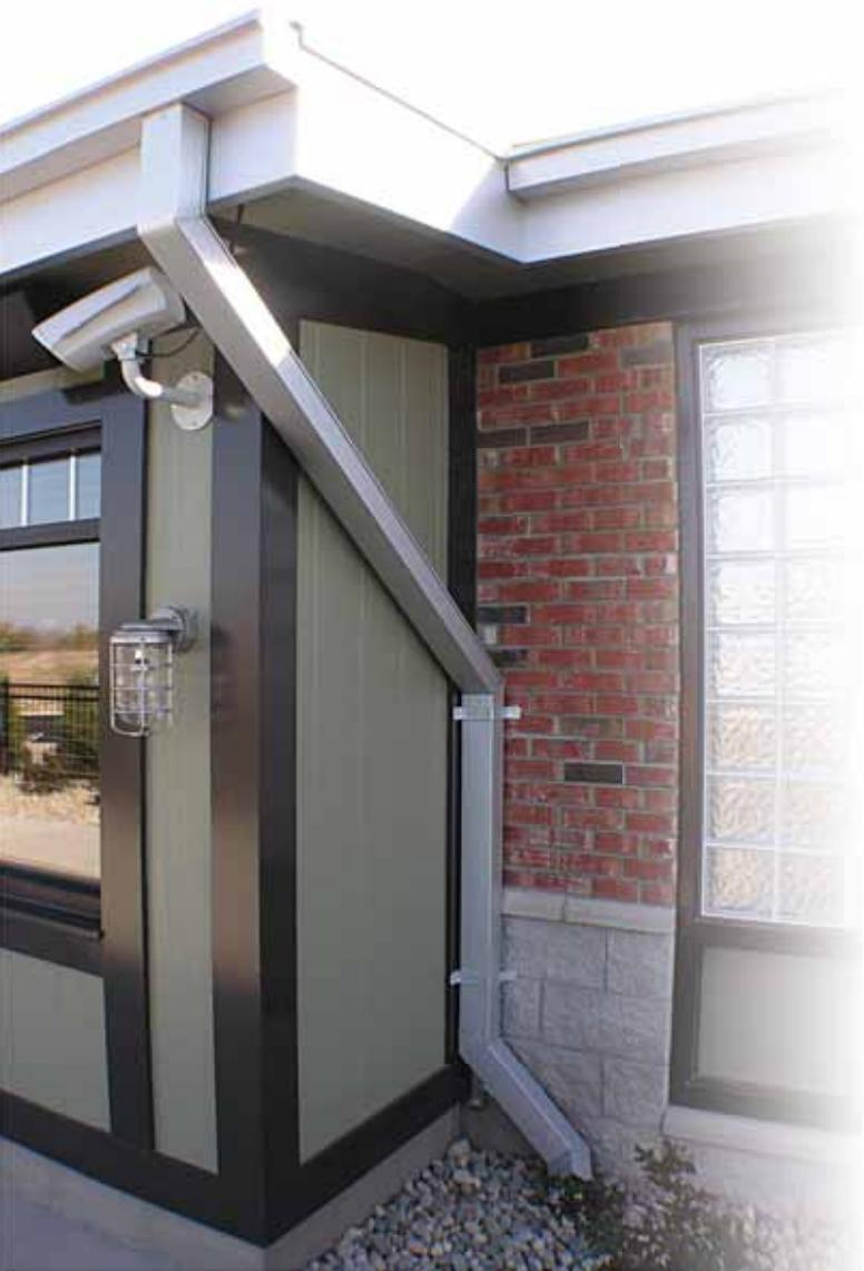
Downspouts are available in a variety of sizes with a traditional closed face or an open face, which prevents blockages from ice and debris.
